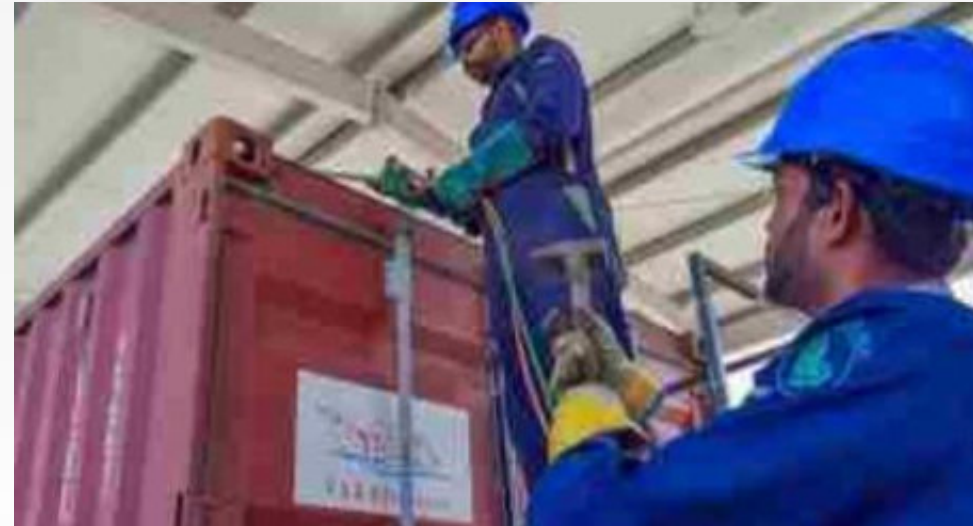
Independent container repair facility of IICL standard
